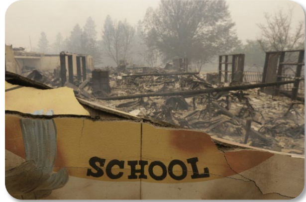
Paradise Elementary School was lost in the Camp Fire. 2018.
